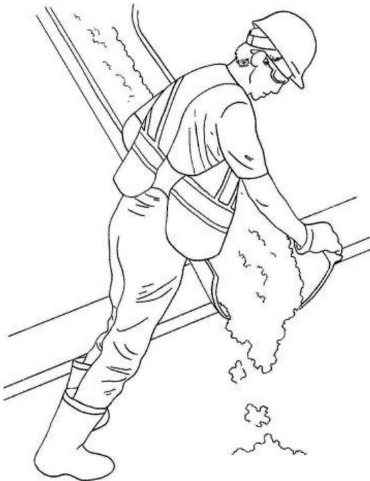
To keep your back out of the job, push and pull the chute with your legs. As you can see here, bridging to the chute with your hips, allows your legs to do the pushing. To pull the chute, step back with one leg into a wide stance, bend your knees, and let your legs do the pulling. Either way you are taking the load off of both your upper and lower back and, at the same time, using the strength of your legs to do the work.
